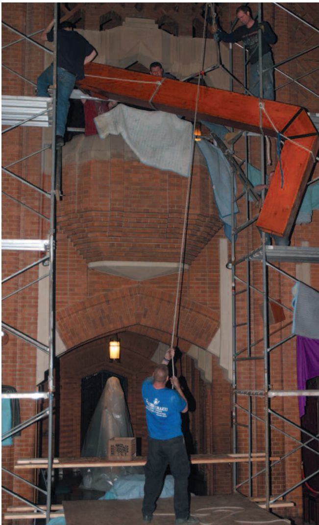
Members from the Organ Clearing House lowering CCC of the 16' Contra Bass to the floor of the church from the organ chambers
